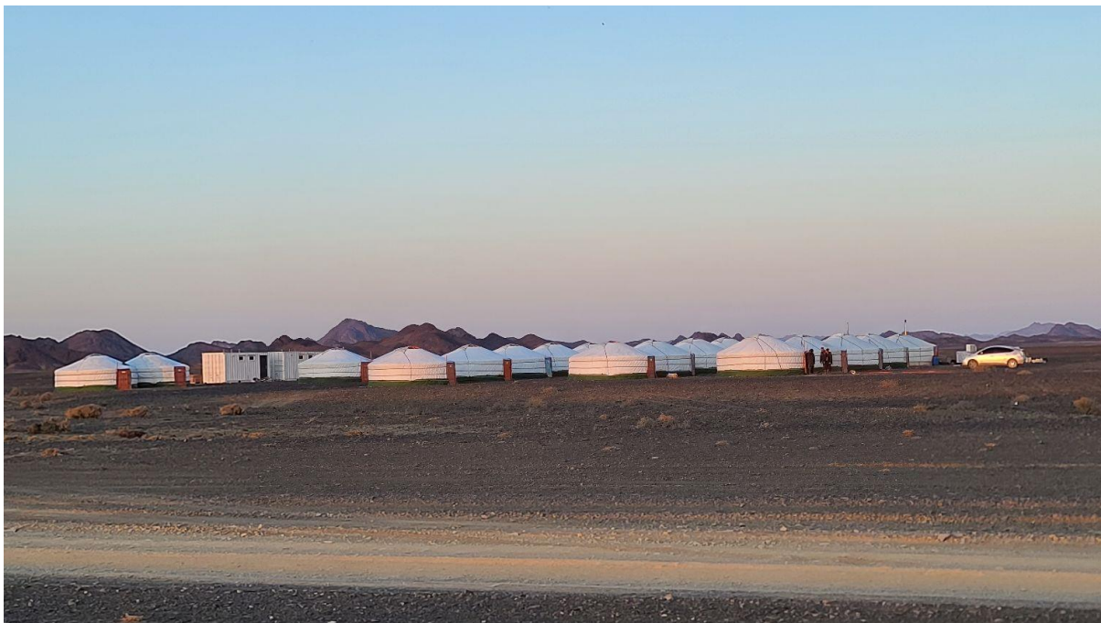
Figure 1 - Exploration Camp for Pilot Well Program Under Construction
