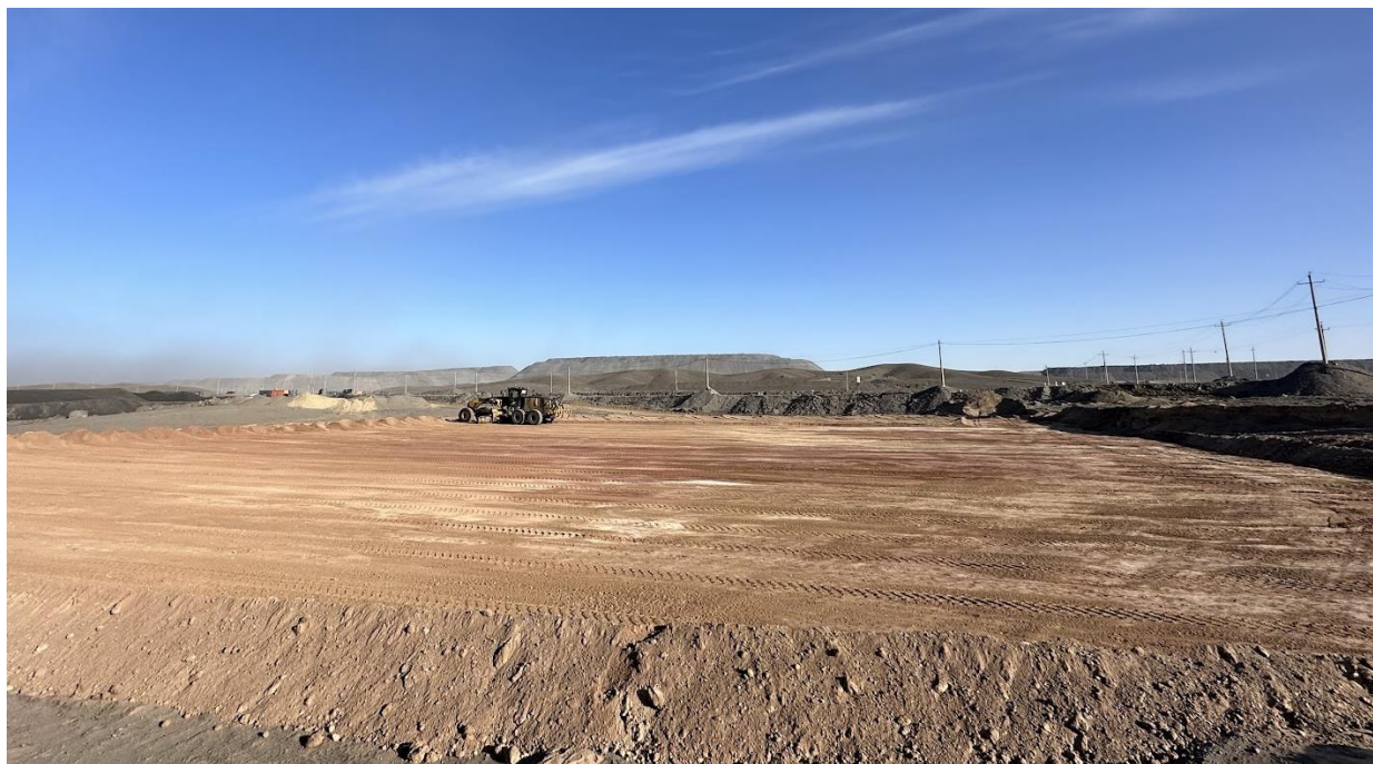
Figure 3 - Preparing Drill Pad for PW-2
