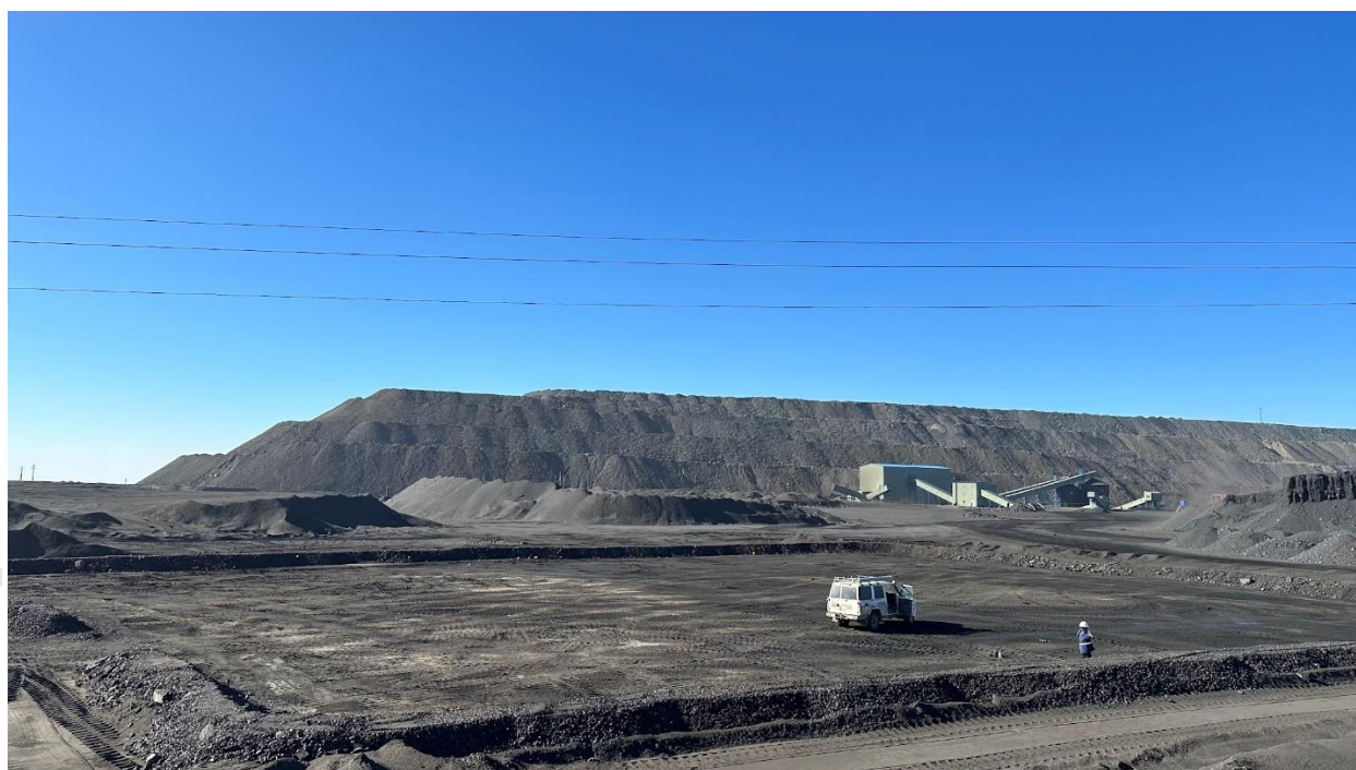
Figure 4 - Drilling Pad for PW-1
