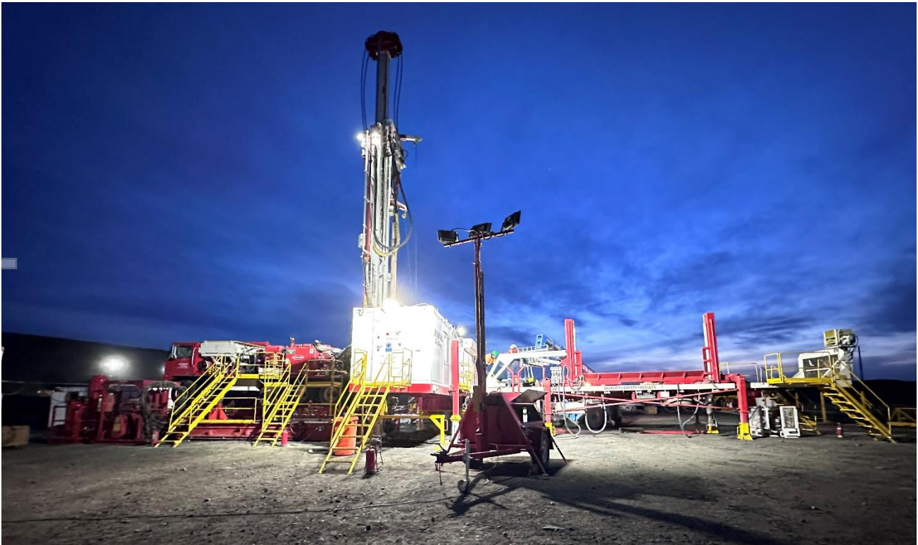
Figure 1 – Major Drilling Rig on location for the Lucky Fox - 1 pilot production well
