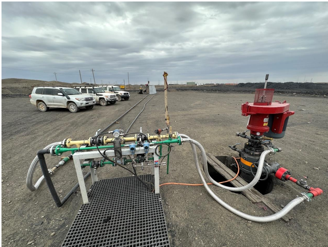
Figure 1 – Completed Lucky Fox - 03 Coal Seam Gas Production Well
