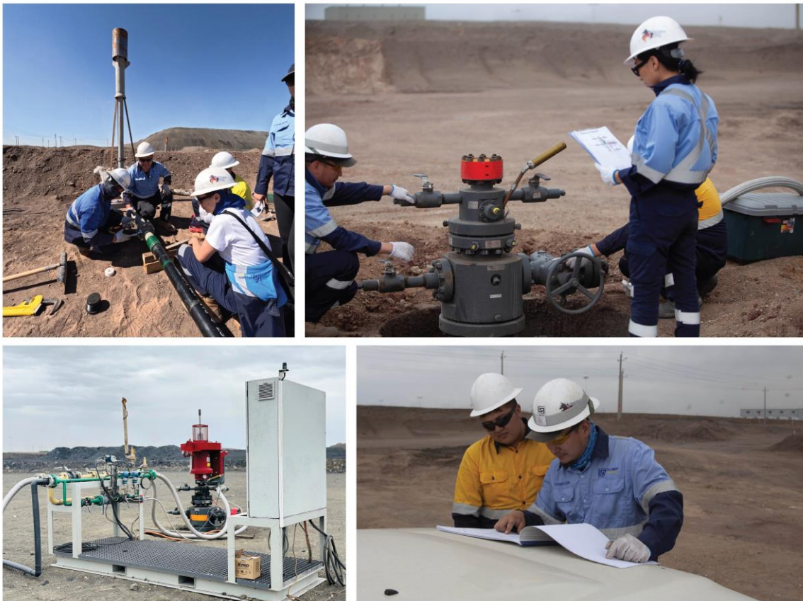
Figure 1 – Commissioning activities at the Gurvantes XXXV CSG Pilot Well Program
